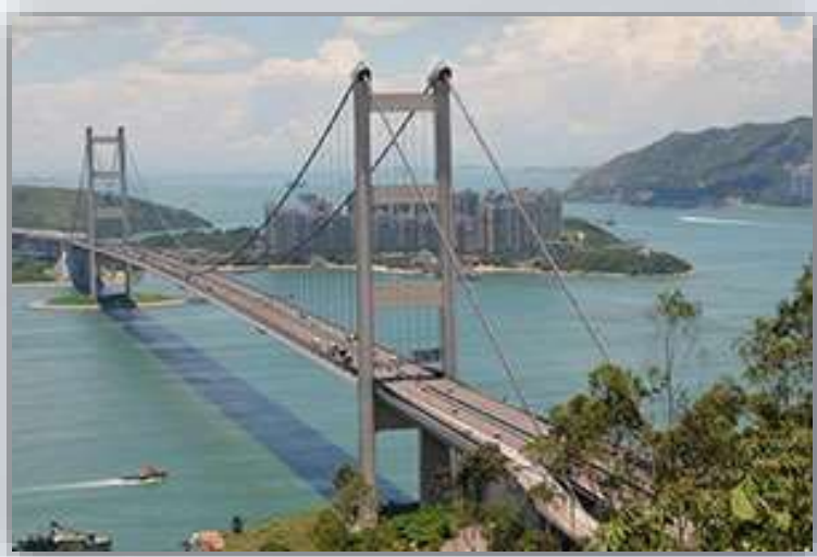
Tsing Ma Bridge
