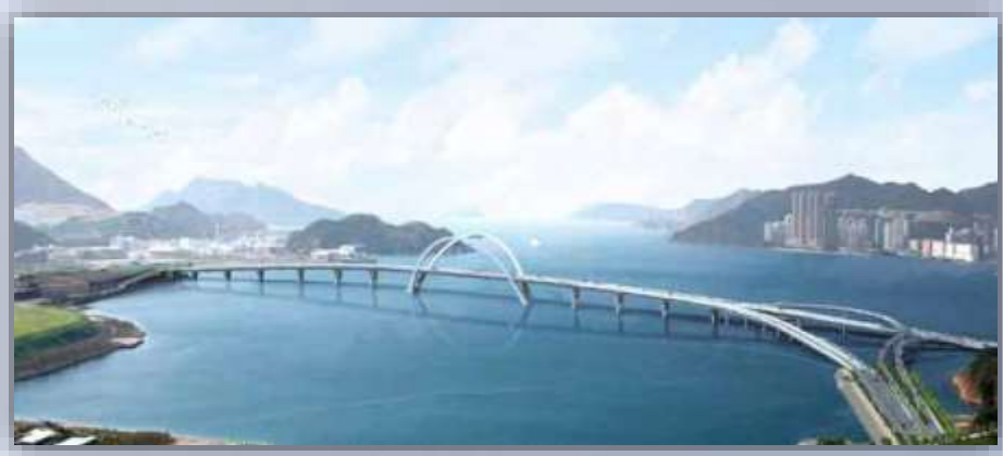
Tseung Kwan O – Lam Tin Tunnel and Cross Bay Link (under construction)
