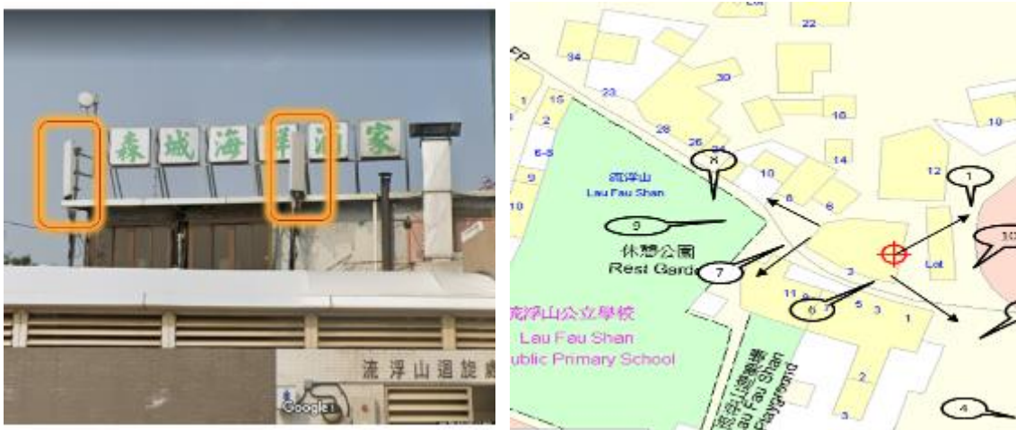
Figure I-6: Photo of Test Site 8 and diagram illustrating the directions of the boresight of the RBS antennas represented with arrows and the measurement points.
