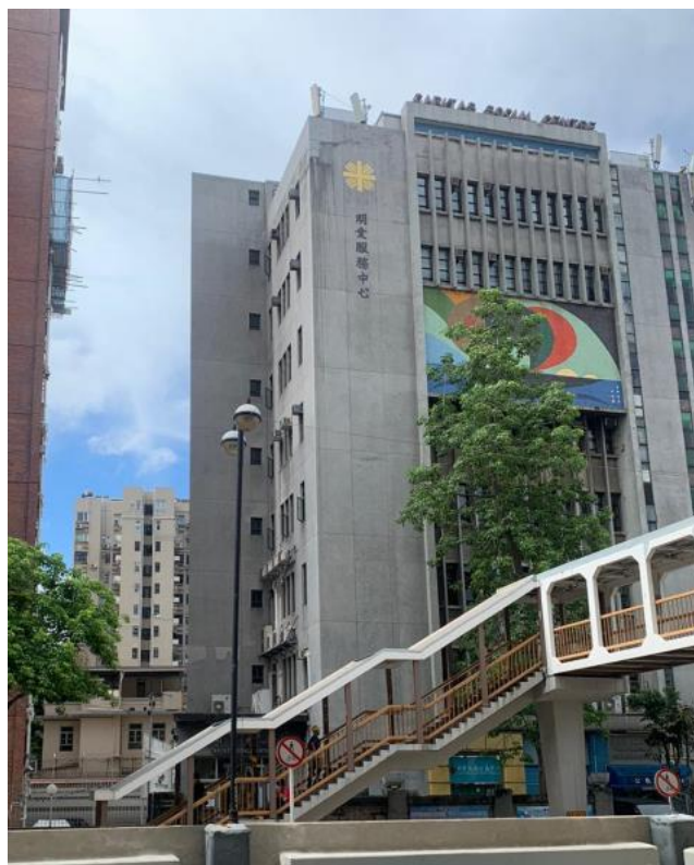
Figure 12 KMB Bus Stop Shelter toward Caritas Social Centre.
